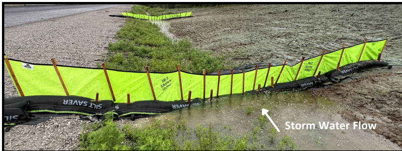
HVDC 24 for flat bottom, trapezoidal ditch
