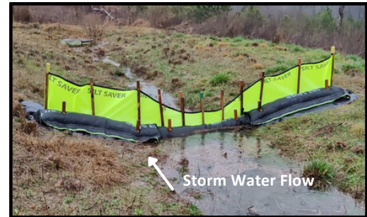
HVDC 14 for V shaped ditch
