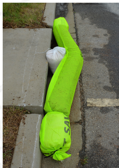
Single SS 300s for 5' inlet opening Use of center weir recommended
